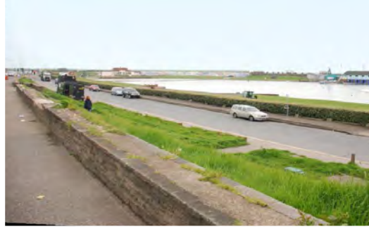
Wharf Road embankment and Hove Lagoon from Kingsway
