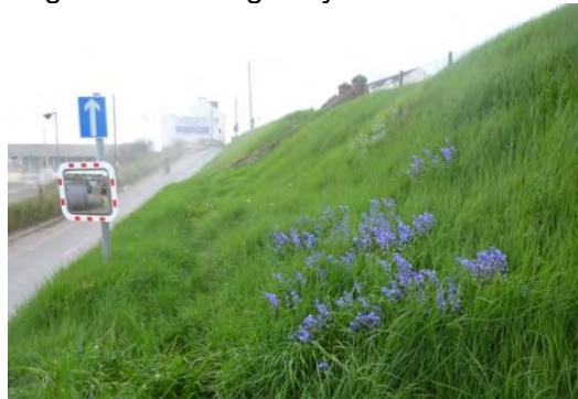
Basin Road North embankment
