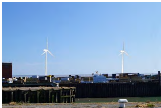
Wind turbines at Outer Layby
